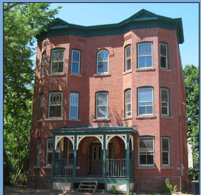
After: CHIF funded the rehabilitation of the building into a two-family home.
