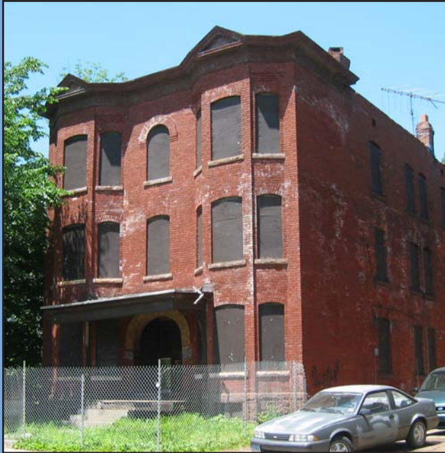
Before: Abandoned apartment building in Hartford, Connecticut..
