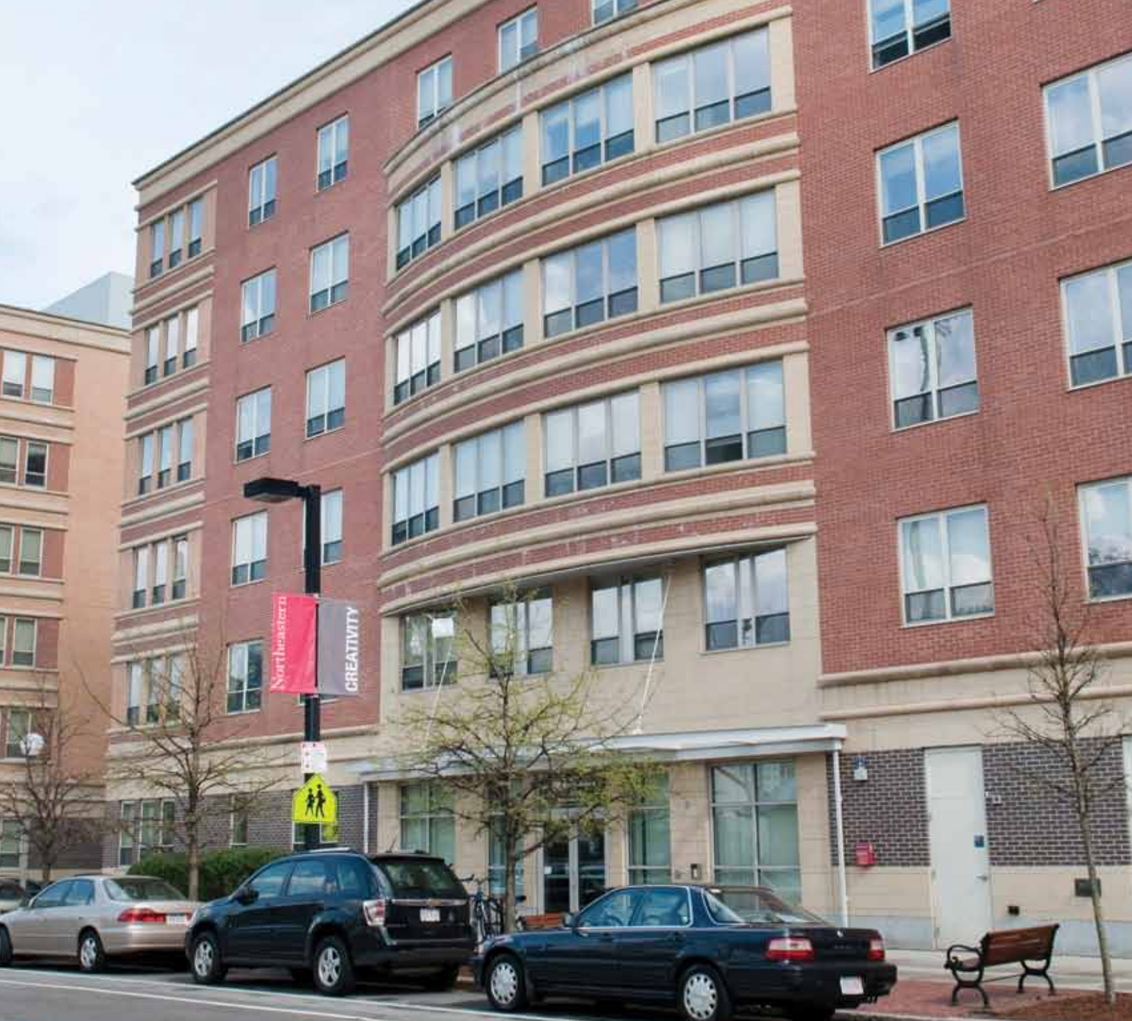
Northeastern University's Davenport Commons project presents a model of community housing. Photograph: Mary Knox Merrill
