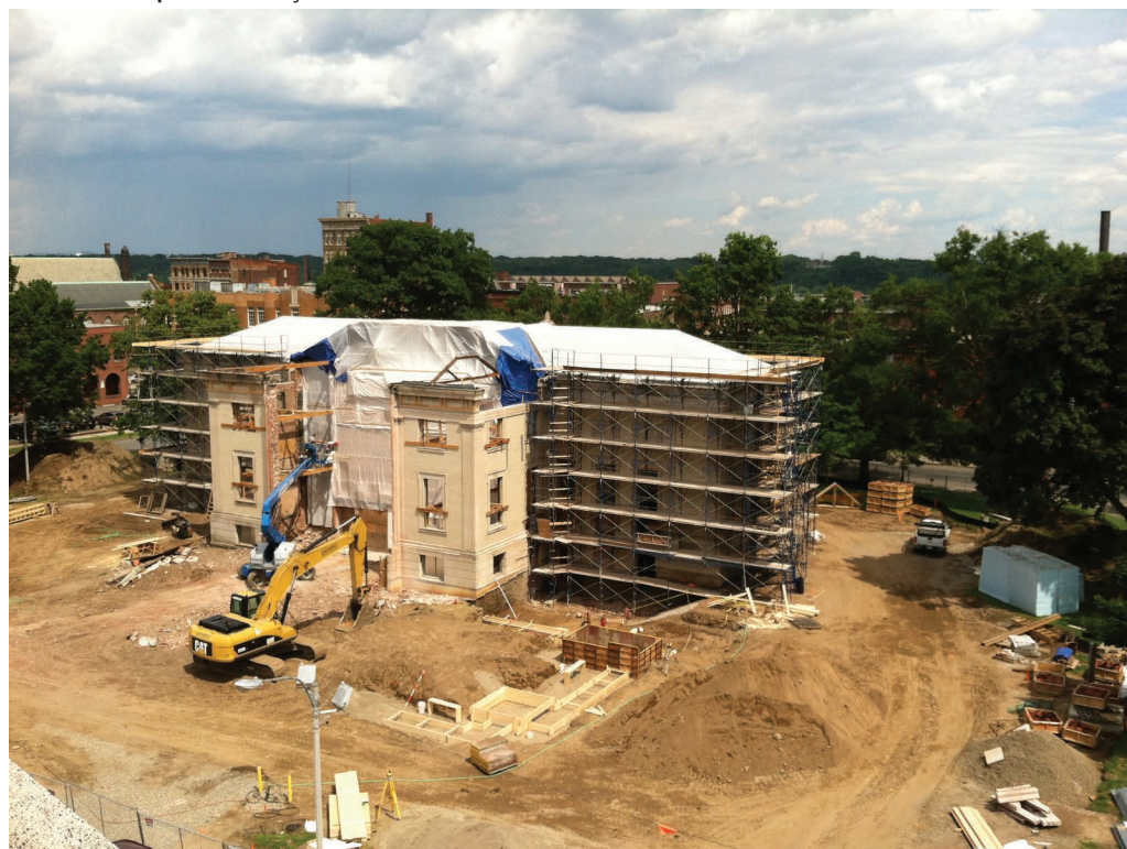
construction photos Sandy Ward
