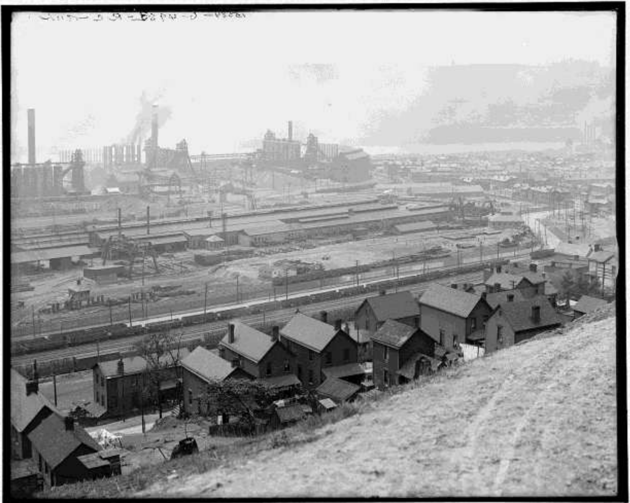
Edgar Thomson Works, Braddock, PA (1908)
