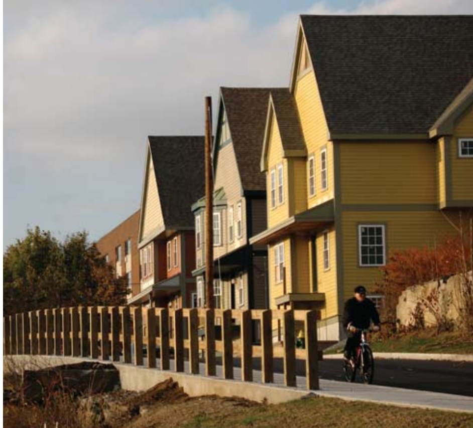
Olneyville Housing Corporation's Riverside Gateway. Photograph: Olneyville Housing Corporation
