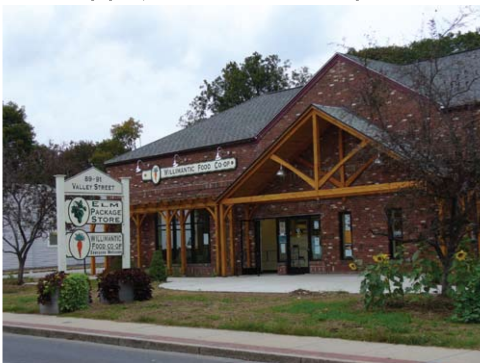
Willimantic Food Co-op has grown steadily since the 1970s and recently moved into space formerly occupied by a supermarket. Photograph: Erbin Crowell
