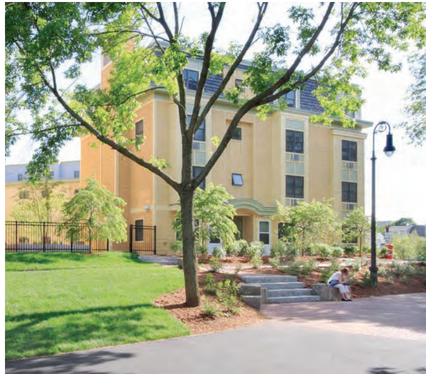
Trolley Square in Cambridge, Massachusetts. Green homes open onto Cambridge Linear Park, a bicycle and walking path.
